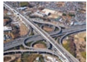
(Photo provided by NEXCO EAST)
