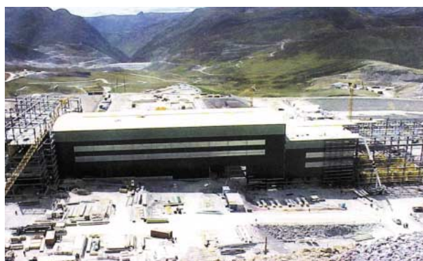
Copper mining development project in Peru
