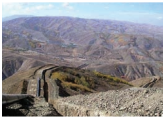
The pipeline passes through highlands in Georgia.
