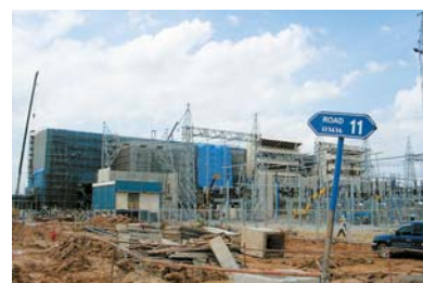
Distant view of power facility No. 1 under construction (June 7, 2006)
