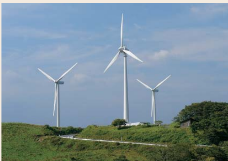
Satomi Ranch wind power generation plant (Hitachi-Ohta City, Ibaraki Prefecture)
