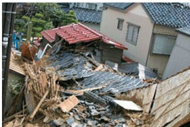
The aftermath of The Niigataken Chuetsu-oki Earthquake in 2007 (Source: Japanese Red Cross Society)
