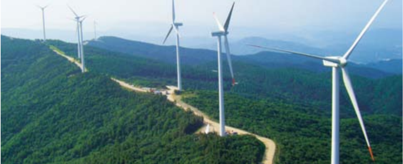
The Taegisan wind power plant has South Korea's leading wind generation capacity of 40 megawatts, supplying electric power that can cover about 25,000 households. The plant is expected to have the effect of reducing CO 2 emissions by about 60,000 tons a year
