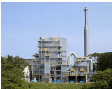
A wood biomass-fueled electric power plant
