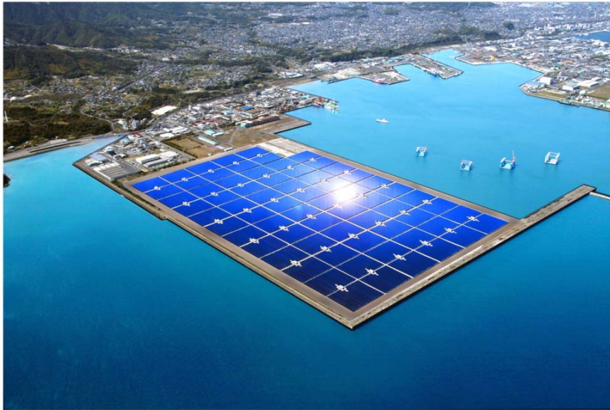
Artist rendering of the completed mega-solar power plant
